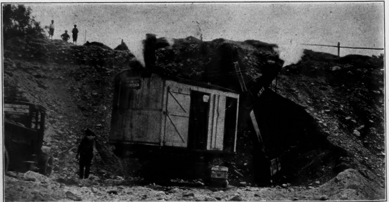
Steam Shovel Loading Material in Pit
